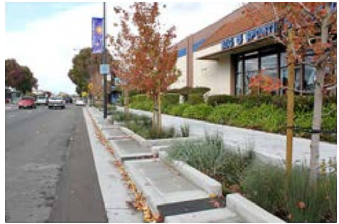
Examples of Green Infrastructure: Left - rain garden, Right - planter boxes in the streetscape.
